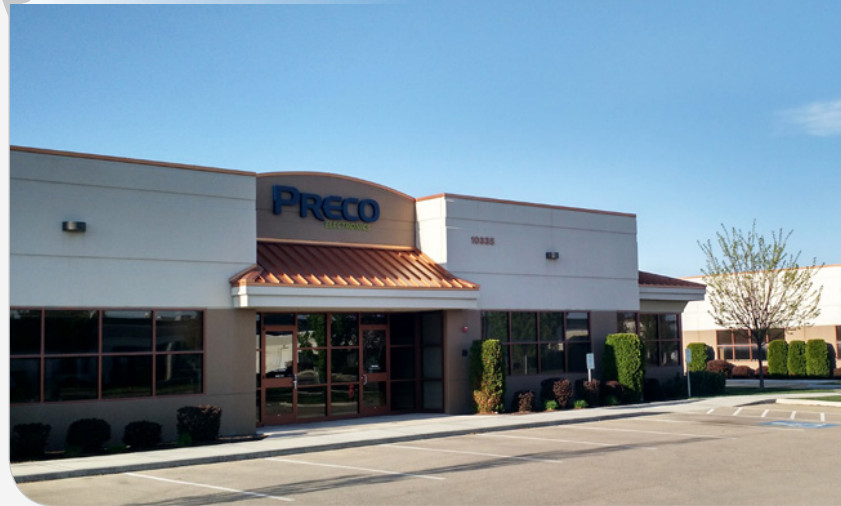
» A variety of horizontal and vertical material changes, reveals, fenestration, and architectural canopies create interest in the building designs from all public views.
