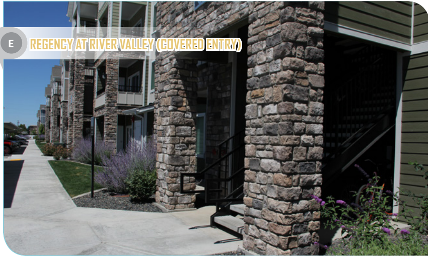
REFERENCES: Natural Appearance, Stairwell
