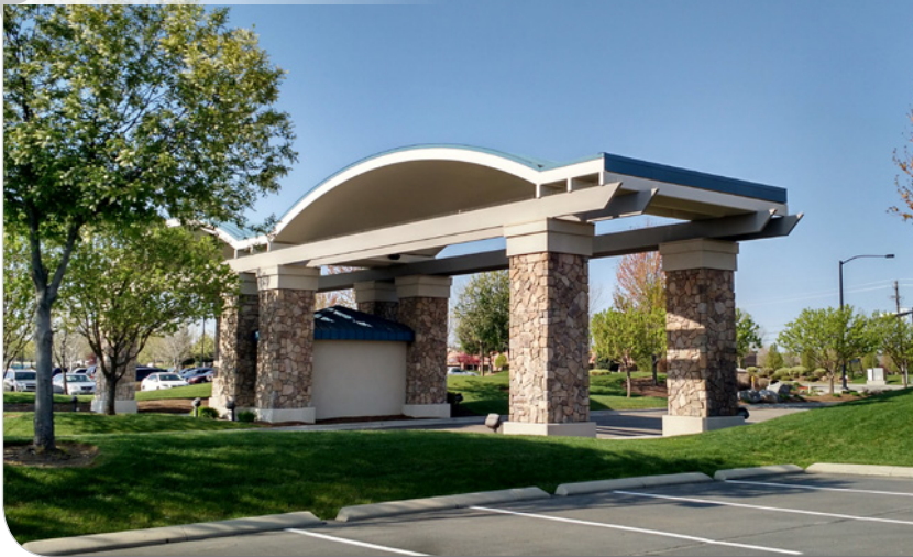
» Unifying architectural element at an entryway to the Silverado business park. Stone and arches are prominent features for many of the buildings.
