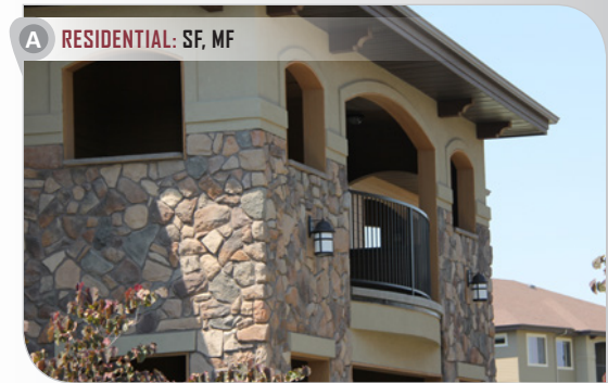
» Stringcourses, lintels, and ledges are all appropriate techniques to transition varying material types into a cohesive design.
