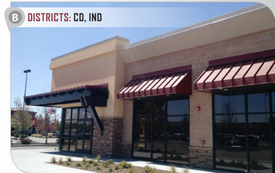
» The building parapet integrates a variety of step-downs, modulation, and material changes to create interest.
