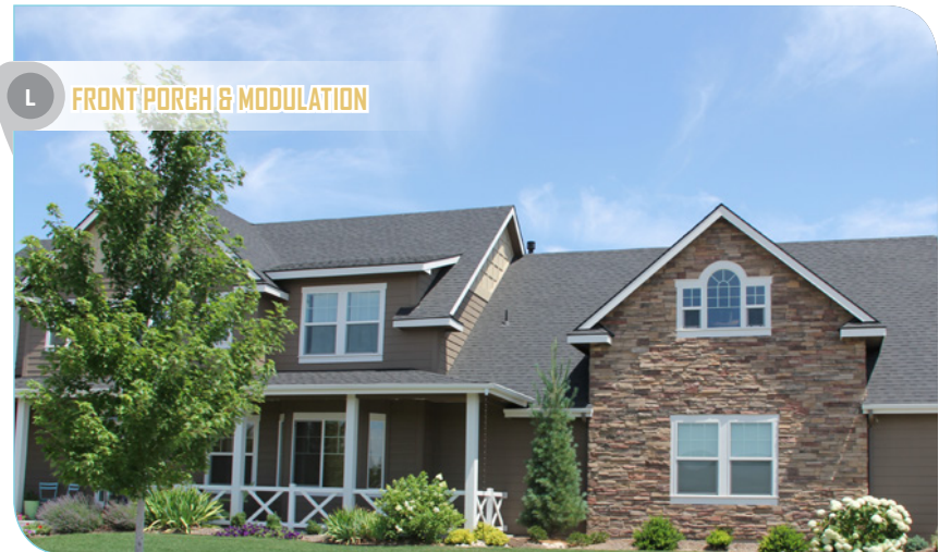
REFERENCES: Porch, Stone and Brick, Stucco
