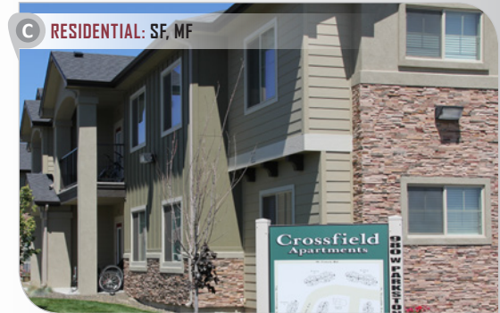
» Windows can be anchored into the building façade through a variety of techniques such as trim, stringcourses, lintels, ledges, railing, or other detail work.
