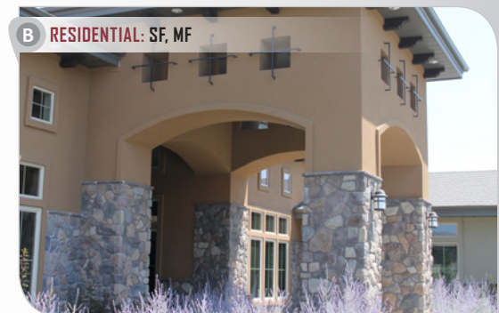
» This prominent entryway feature makes use of columns with stone accents, ledges, portals, recessed lighting, and other architectural features such as corbels and tracery like features.
