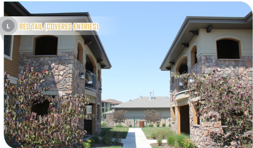
REFERENCES: Eaves, Railing, Soffit, Stone and Brick
