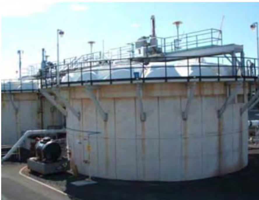
Figure 4-10. Covered gravity thickener
